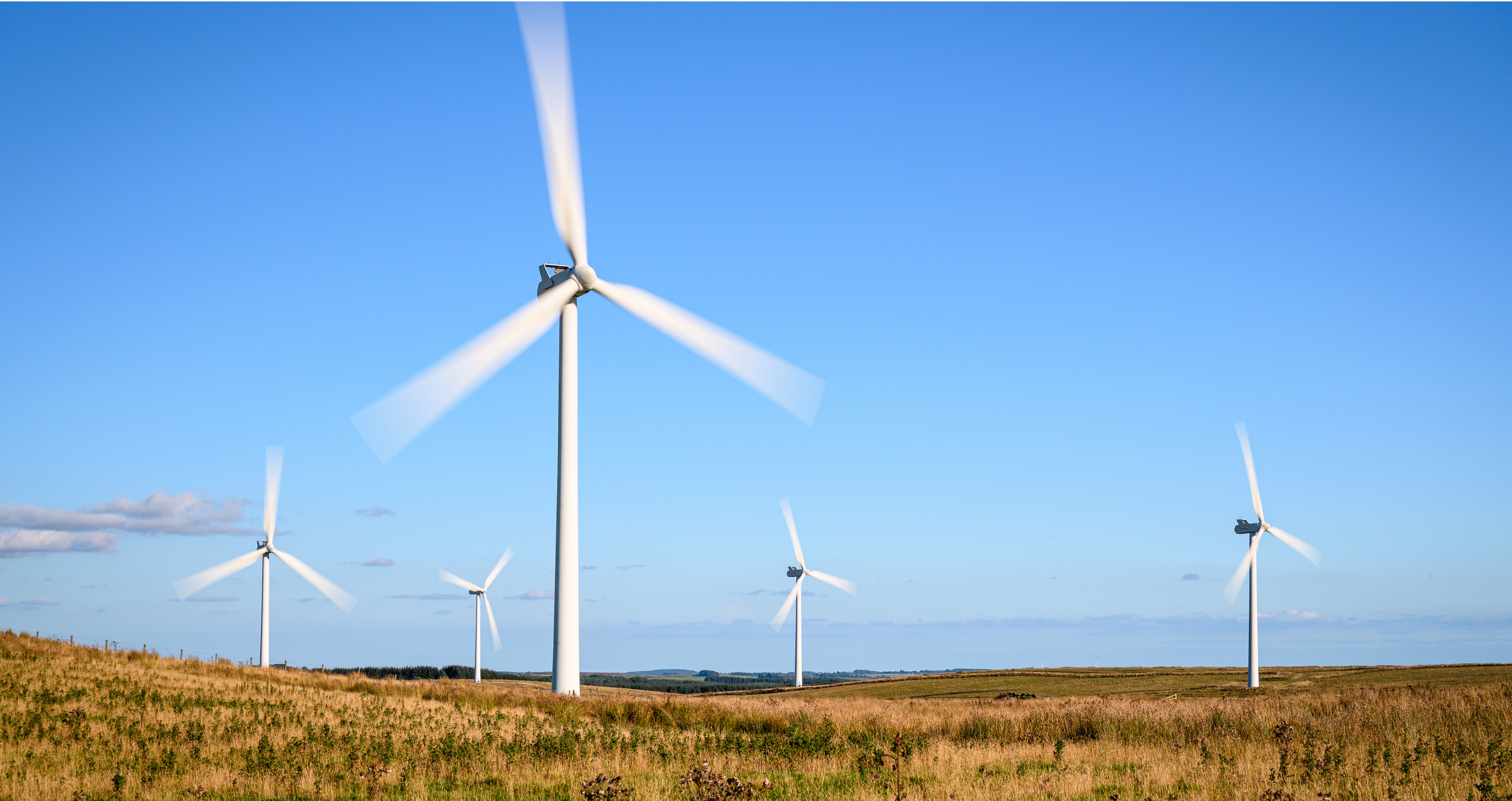
Image of a typical Energy Park for indicative purposes only
